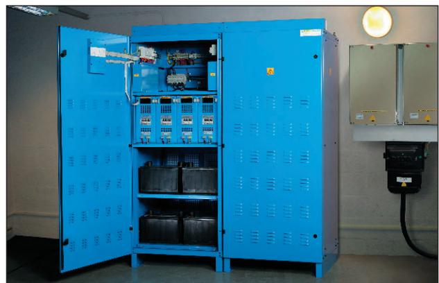
EMEX Power cabinets require no side ventilation therefore are easy to install in virtually any plant room
