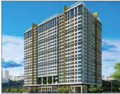
Project THE GALAXY RESIDENCE Investor NOVALAND
