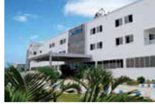
Rudrapur Plant (Green Building)
